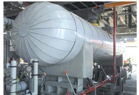
Vessel Insulation
